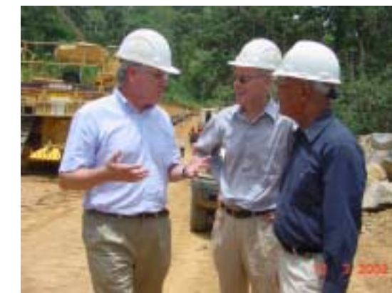
Mr. Michel GALLET, the General Manager of COTCO (on the left), explaining the different steps of laying the pipeline
