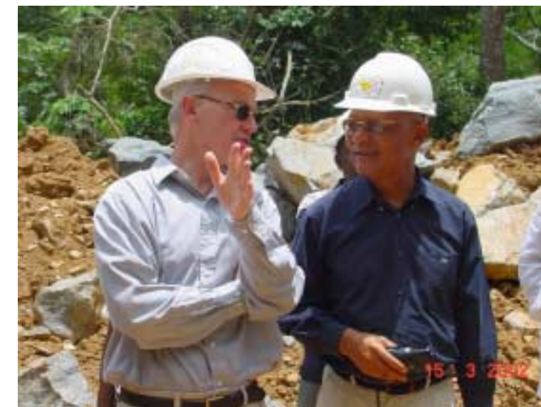
Mr MOUDIki (on the right) and Mr MADEC, on the Bipindi Landseasement, very impressed by the progress of construction work
