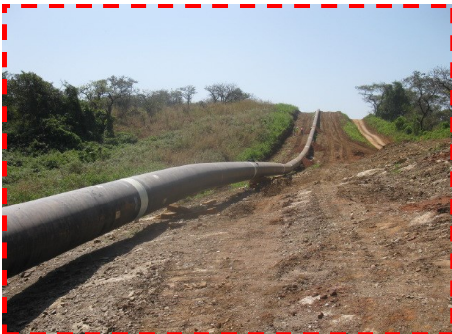
The inner face of the Pipeline has been cleaned
