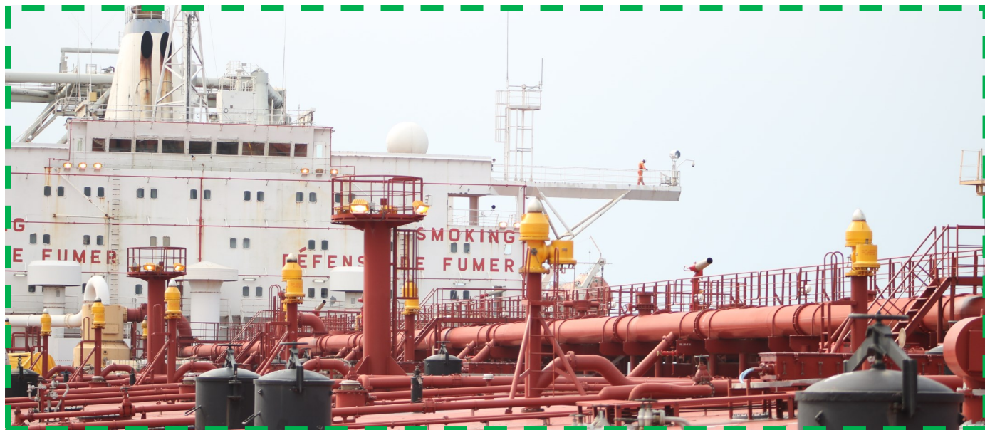
Terminal KK1 has been inspected
