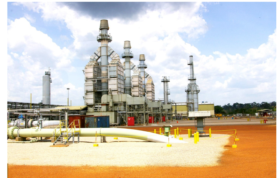
Belabo Pumping Station was inspected
