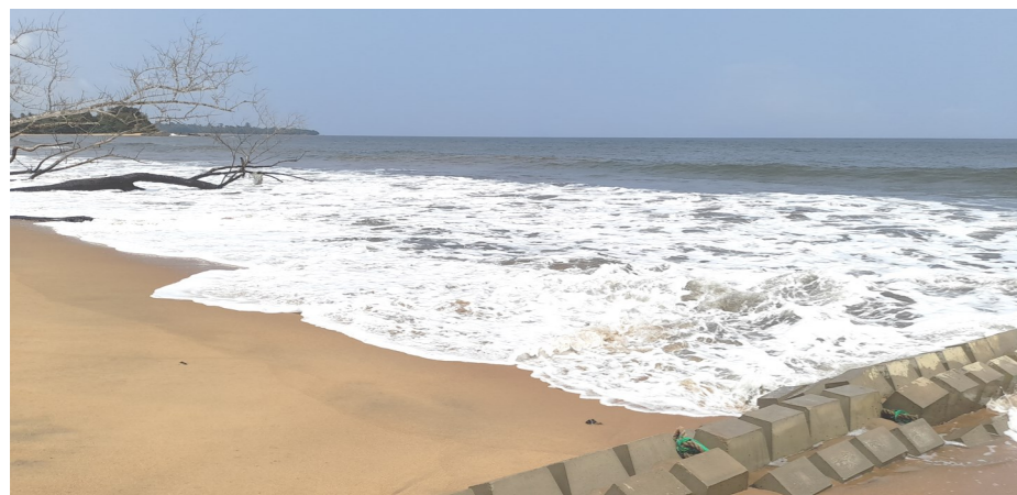
The area of erosion after repair
